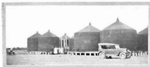
Resonians inspect Messrs. Hepworth's Oat Silos at Woomelang.
