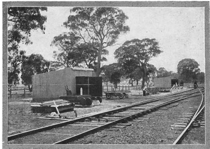
Permanent Way Ganger's Tool House. Exterior View.
