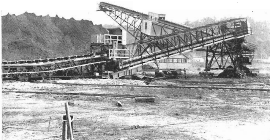
Removing Overburden at Yallourn
