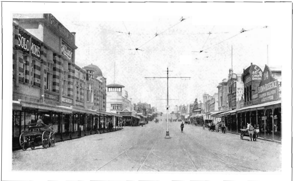
Moorabool Street, Geelong.
