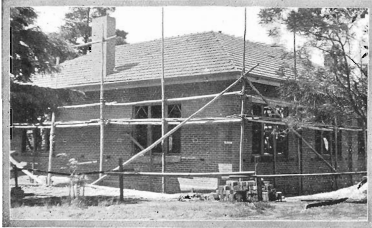
New Institute Building being erected at Bendigo.
