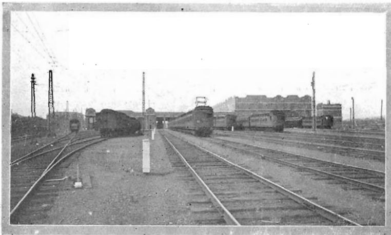
View of Jolimont Workshops, showing electric train and locomotive
