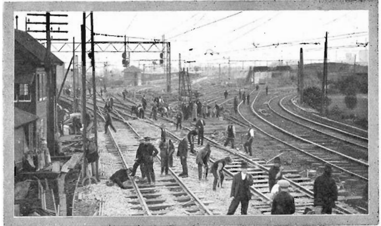
General View of Reconstruction Operations.
