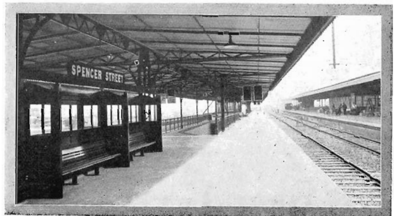
General View of Platforms
