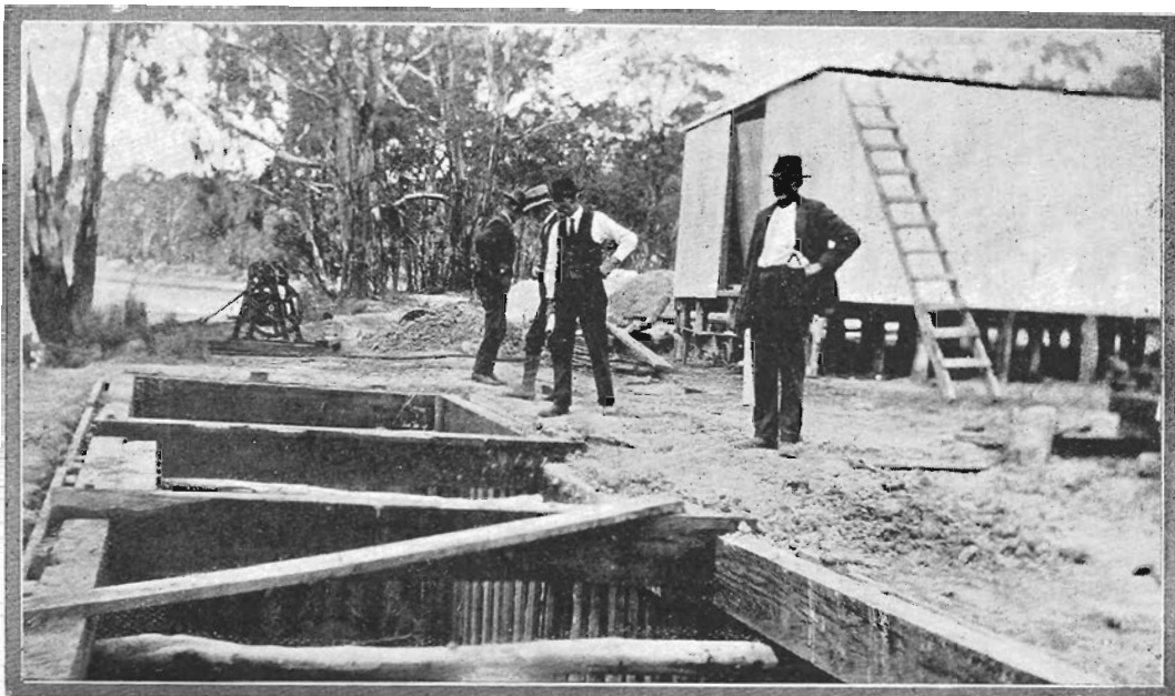
Bridge over Murray at Gonn Crossing. Commencement of Work.
