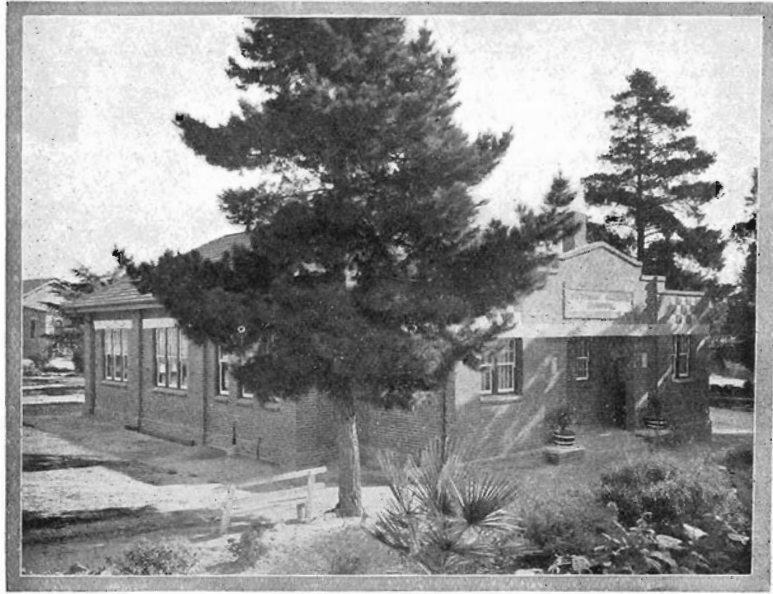
Front View of New Building.
