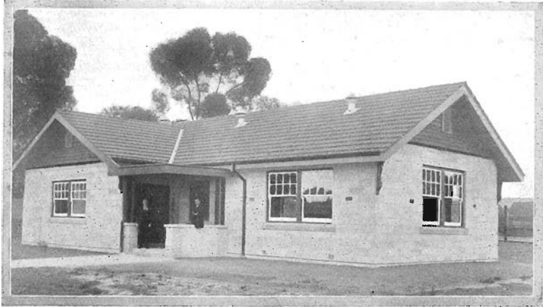
North view Benalla Institute Building.
