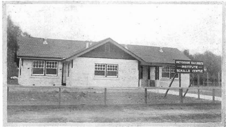
Front view—Benalla Institute Building.
