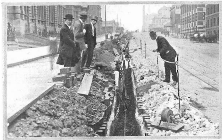
Laying 20,000 Volt Cables in Trench.
